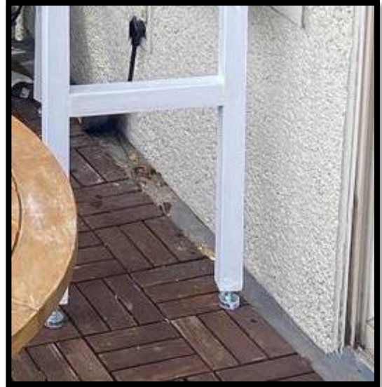
Figure 12: Leveling Furniture Feet Installed
